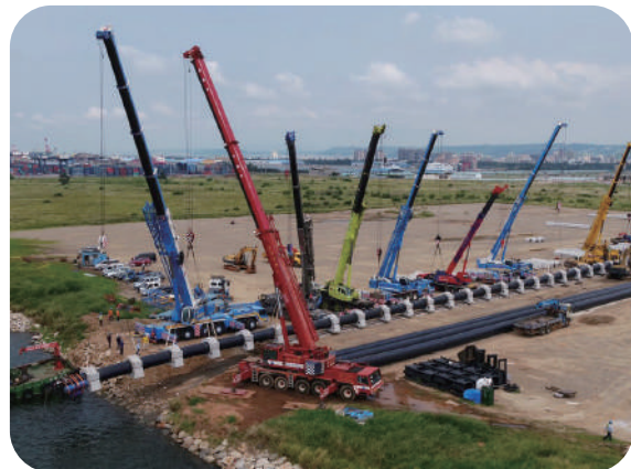
■ New seawater pipes of Taiyen
